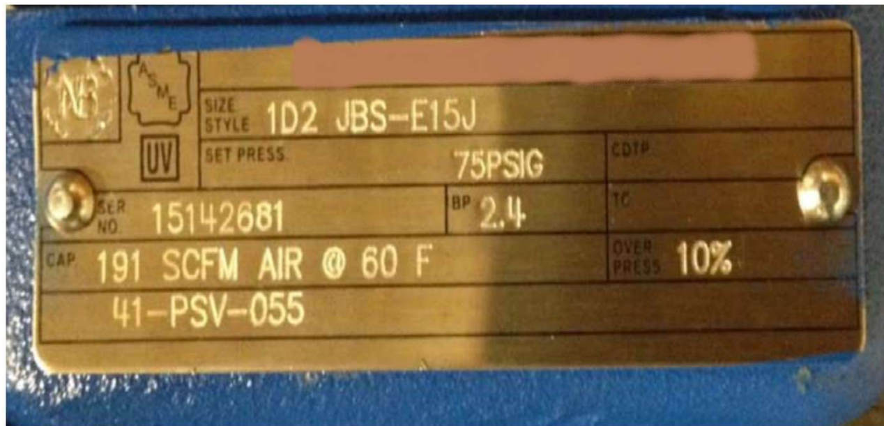
Figure 40a—Identification Tag for Pressure-relieving Device (pre-2013)
